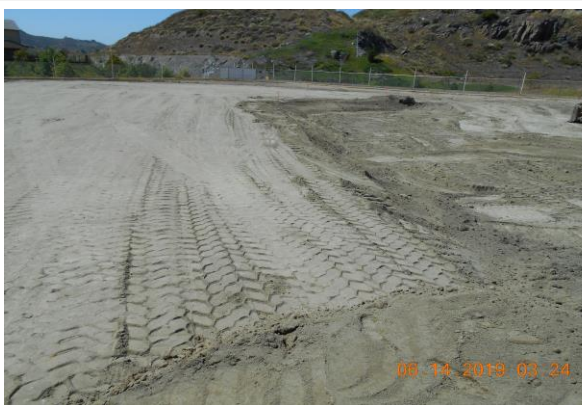
Compaction of Building Pad
