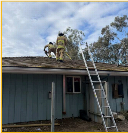
Ground ladders and vertical ventilation.
